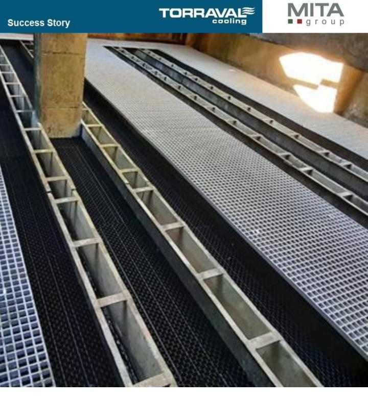
In addition, **drift eliminators** were replaced and tramex-type **working platforms** were installed to facilitate the **water distribution system** cleaning and maintenance tasks, allowing access to any point on the cooling installation surface.
