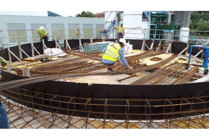
The concrete upper part of the field erected cooling tower consists of a platform where the mechanic equipment is pinned. In the center, we place a GRP diffuser. In all the length of the side of water entry, we find the reinforced concrete major collector.
